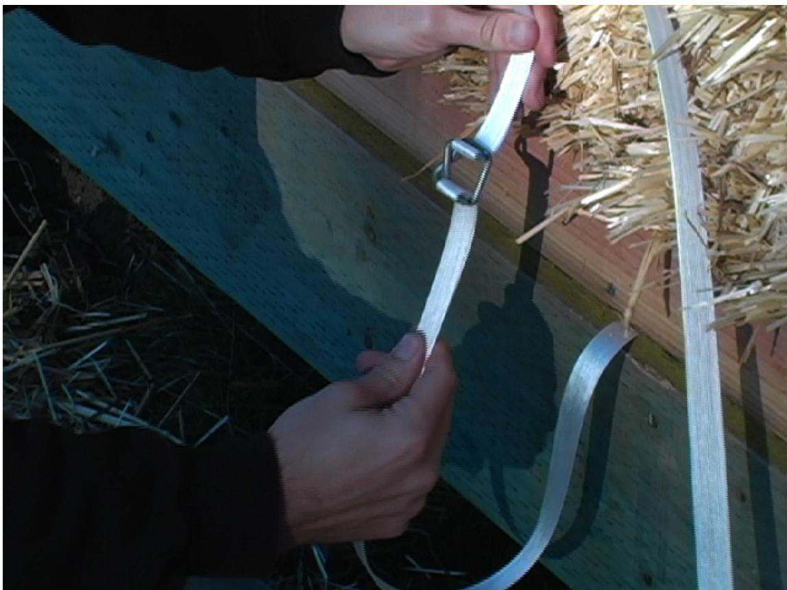
two courses of bales then cut two sections of cord strapping that are long enough to go around two courses of bales and drape them on top of the first two bales. Place a 2x4 block between the framing members and push it as far down onto the top of the bale as possible. Toe-nail the blocks into the wall framing, place the next two courses of bales on top, wrap the strapping around the bales, and then tighten the cord strapping around the blocking and bales.
