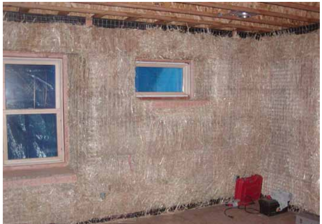
Welded wire mesh applied over the bales and ready for plaster.
