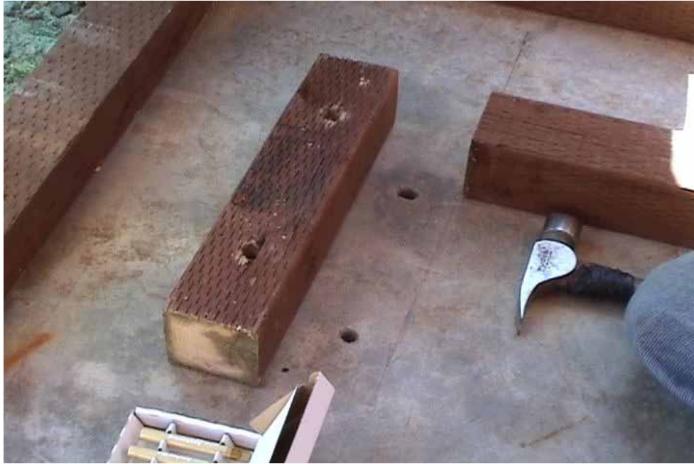
Structural, interior toe up ready for installation
